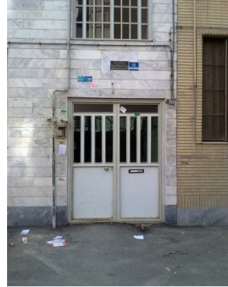
Figure 2 - Straight forms in a district 12 House,
